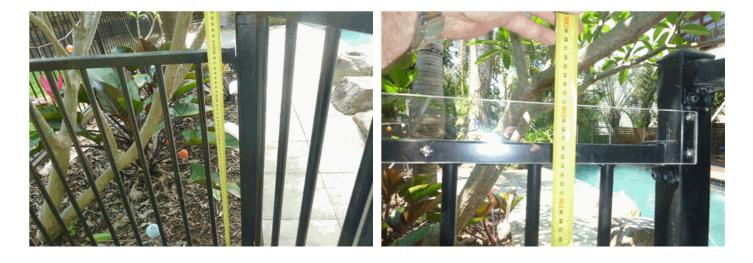
4) Identify which side of fence for effective NCZ NCZ for this pool is on the outside of the Barrier.
