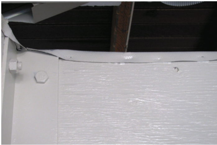
Photo 4: Flashing installed over H3 LVL beam under a deck.
