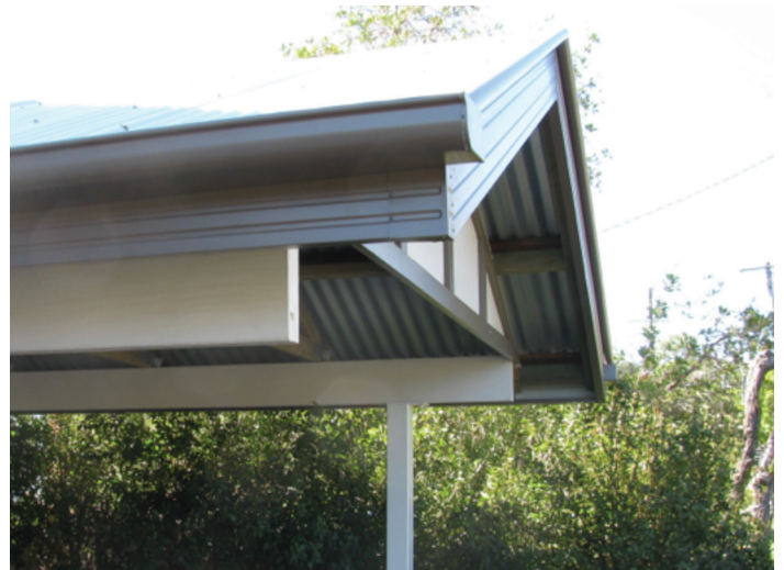
Photo 3: Adequate overhang and quality pale coloured paint system provide good protection to end grain and sun exposure.
