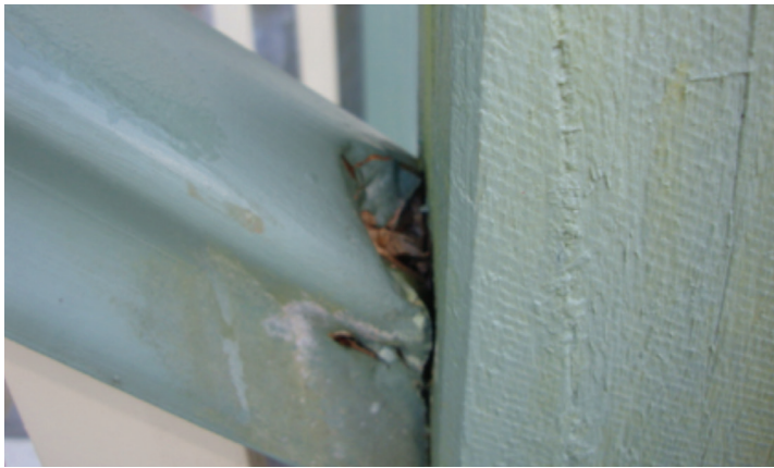
Photo 1: - Avoid premature failure by applying supplementary preservative and oil-based alkyd primers on all cuts, notches, holes etc.
