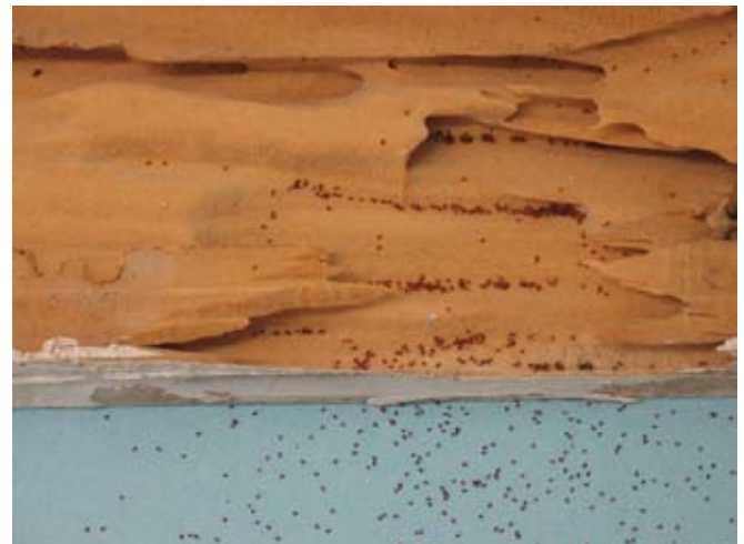
Figure 3. Galleries and frass in a section of pine.
