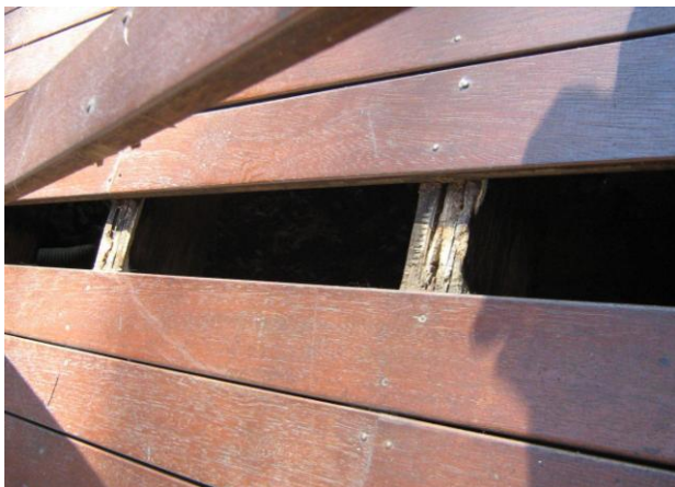
Removing this decking board has revealed a decayed joist
