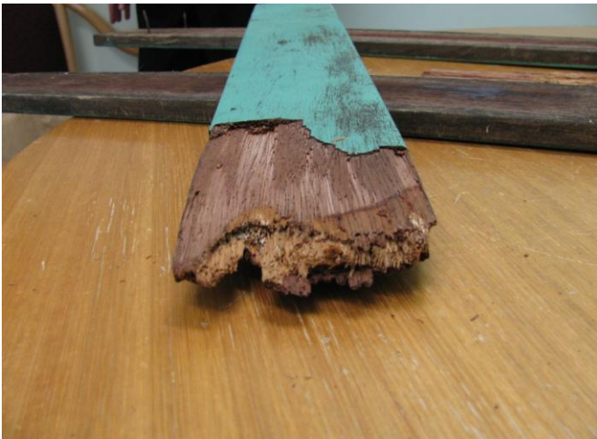
One of the decayed decking boards from the accident.
