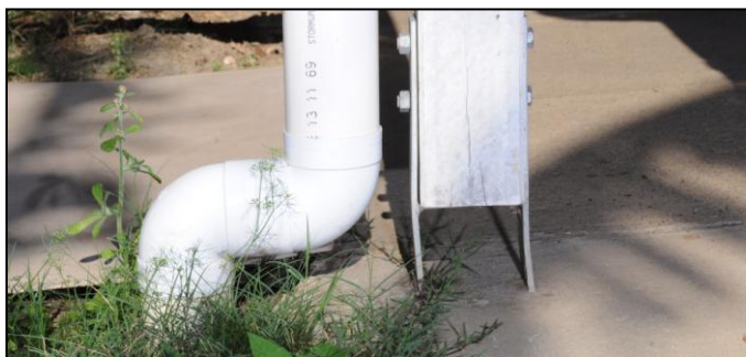
Inspect post brackets for bending or stressing
