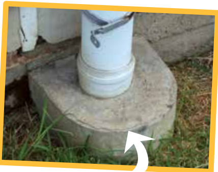
DT surround (disconnector trap)
