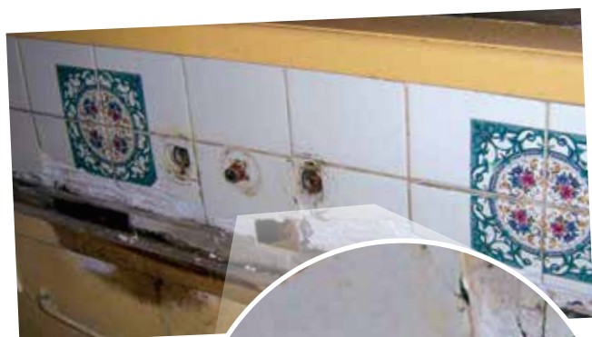
Ceramic tiles on asbestos sheeting
