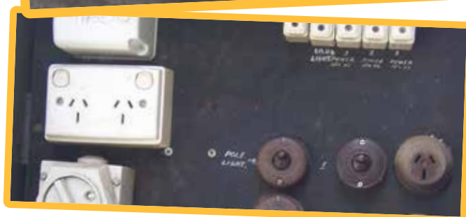
Zelemite backing board to an external switchboard
