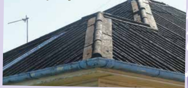
Super six roofing ridge capping and guttering
