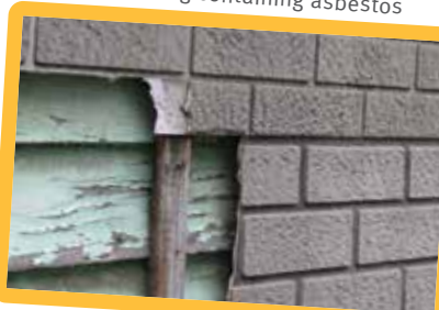
External cladding containing asbestos
